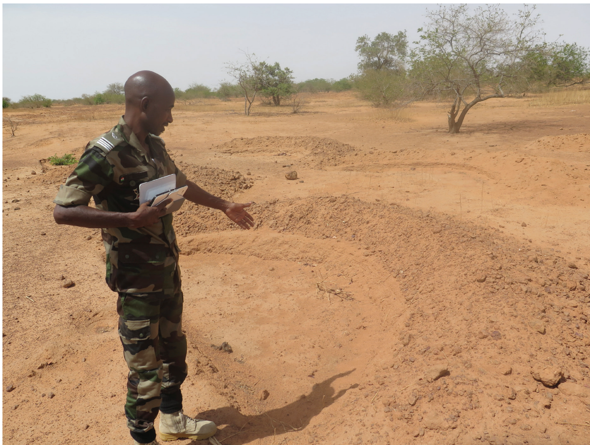
Half-moon water retention technique being implemented in Sokorbe, Niger; Nasser Alqatami, @ LoCAL-UNCDF
