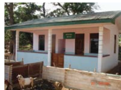
A Clinic Post in Bauro village, Lospalos Sub-District has been well maintained, and the community built a fence to prevent animals from entering the building
